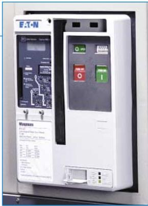
Safety is enhanced by the through-the-door design that provides for three breaker positions with the door closed: connect, test, and disconnect.
