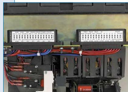
Positioning of the secondary contact subassembly is dedicated for installation, maintenance, and testing. Top view shown with breaker cover removed, bottom of photo is front of breaker.
